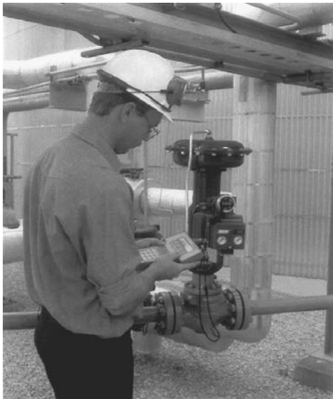
Figure 6.2 Two-way communications link with a digital positioner, using a HART Handheld Communicator. (Courtesy of Fisher Controls International)
