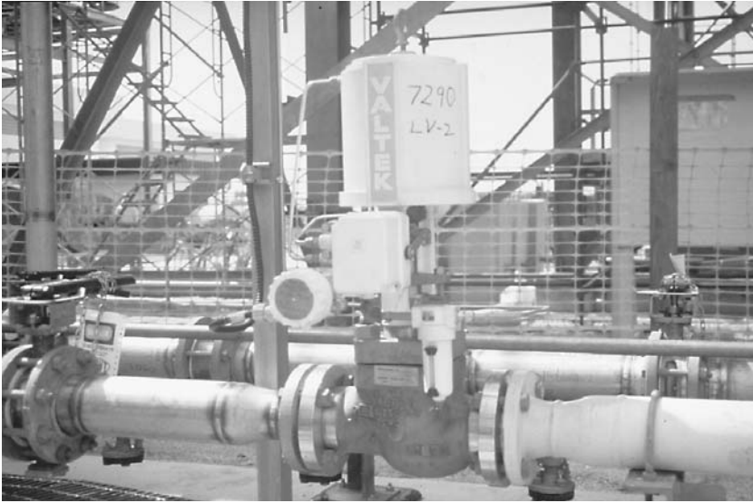
Figure 5.12. Piston cylinder actuator. (Courtesy of Valtek International)
