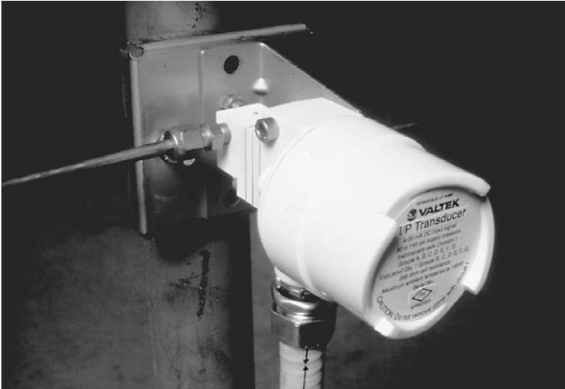
Figure 5.63. Transducer separately mounted from actuator. (Courtesy of Valtek International)
