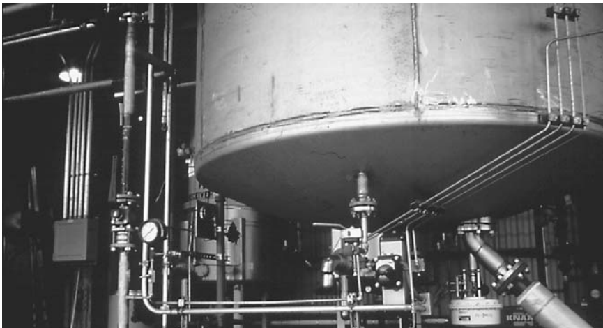
Figure 1.2 Tank bottom valve used in a steel processing application. (Courtesy of Kammer USA)
