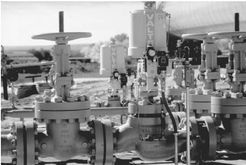
Figure 1.9 Wedge gate valves used in a blocking service to bypass general service control valves in a gasification process. (Courtesy of Valtek International)
