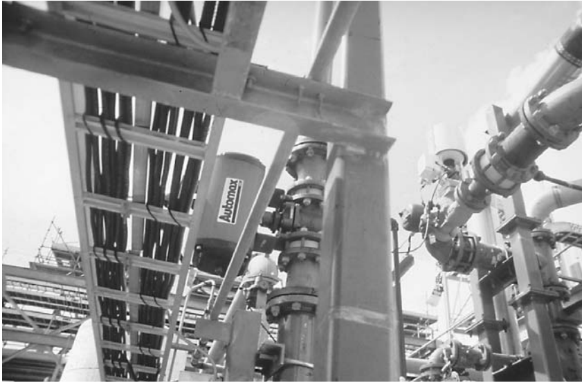
Figure 1.3 Quarter-turn plug valve with rack and pinion actuation system in chemical service. (Courtesy of Automax, Inc. and The Duriron Company, Valve Division)
